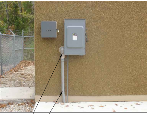
LB PROVIDED AND INSTALLED BY SHELTER MANUFACTURER POWER MUST BE RUN INTO THE SHELTER THROUGH THE LB CONDUIT, NOT THROUGH THE DISCONNECT BOX
